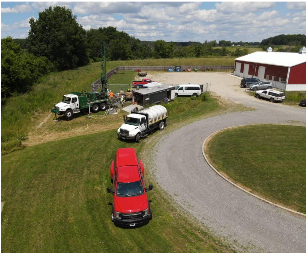
Coring, monitor well installation, purging well
