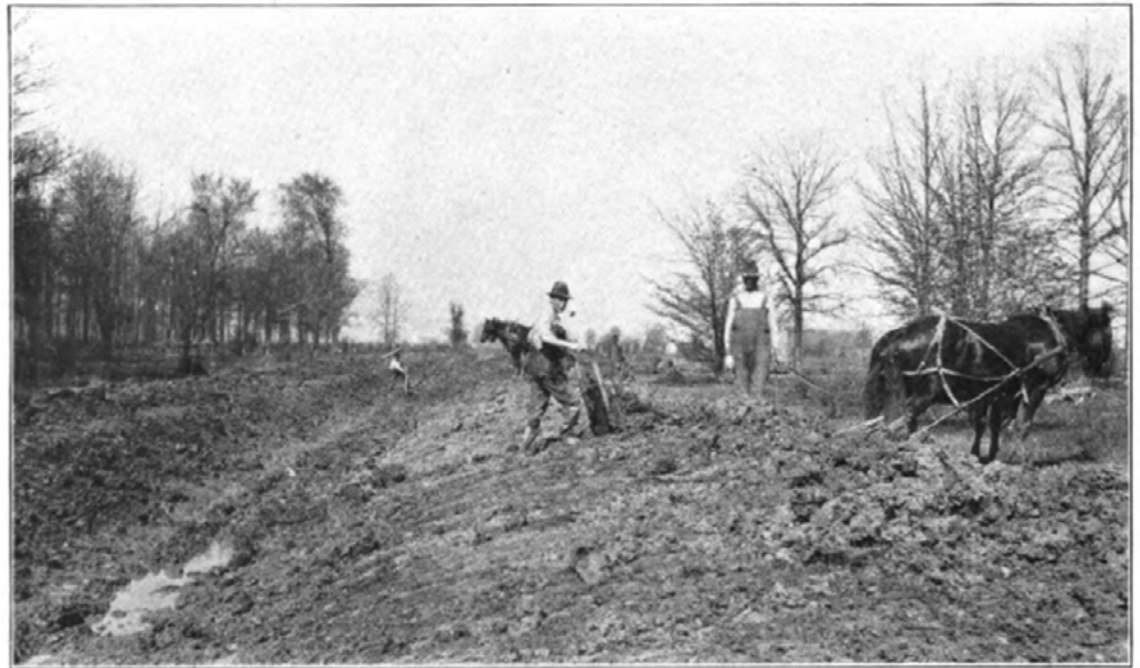
CONSTRUCTION OF OPEN DRAIN, THREE FEET BOTTOM WIDTH, FOUR FEET DEEP WITH BOARD SCRAPER AND TEAM
